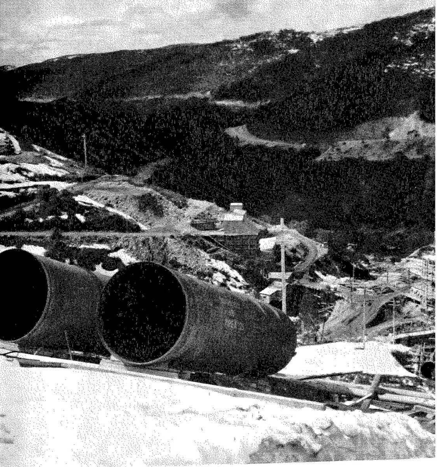
Looking on to the Munyang Power House. Roadway in distance leads to the Snowy River Valley.
