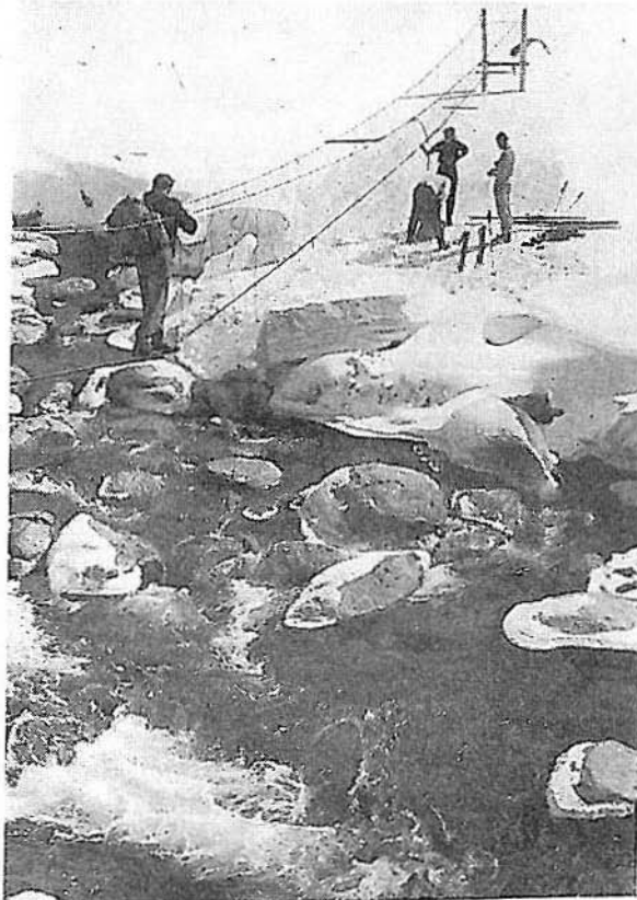
JIMMY'S BRIDGE. The nervous preferred rock-hopping, but many crossed the Snowy near Foreman's Hut in this way. S.T.A. members Jimmy Walker, Ian Curlewis and Margaret Anton built this 50-yard suspension bridge during the Easter week-end, 1954. For '55 the bridge will have planks between the two bottom wires, making tightrope walking unnecessary.
