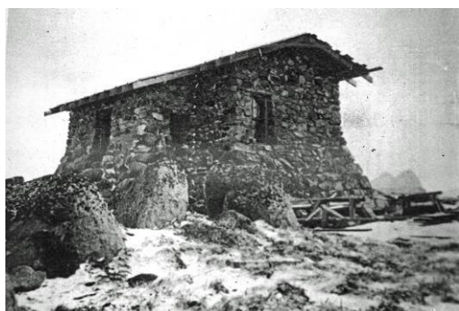
Seamans Memorial Chalet under construction March-April 1929 (unknown, from CMP 1989)
