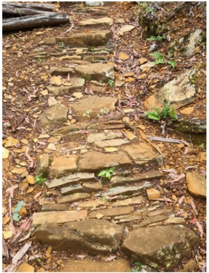
Higgs Track with traditional Scottish stone paving
