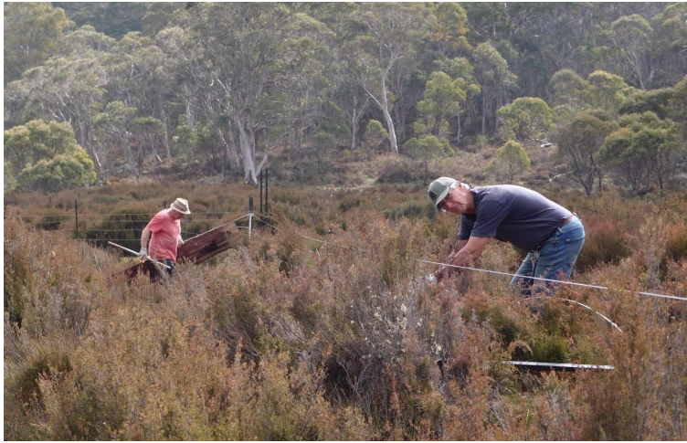
Jim and Murray building the horse exclusion fence at Tin Mines 24 April 2023
