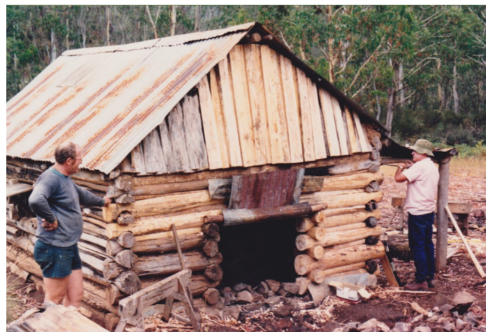
John Hamilton at Vickers showing repaired chimney - 1988 Khuts.org
