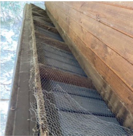
Above: repair to net
