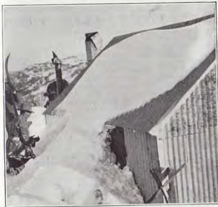
THE PARTY DIGGING THEIR WAY INTO TIN HUT.
