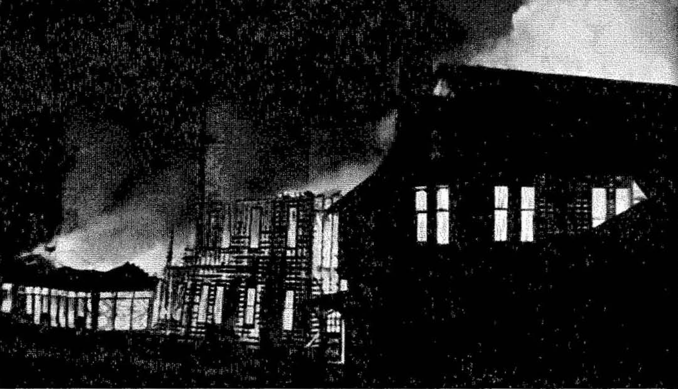
The Fire from the North Side.
