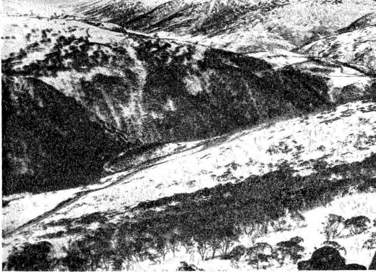
View from Blue Cow Mountain showing roadway to Guthega, Snowy River, Munyang Pipe Line, Munyang or Whites River, Disappointment Spur and Mt. Gungahen (6790 feet).
