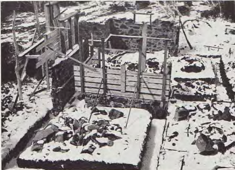
Building of the new Hut in progress.
