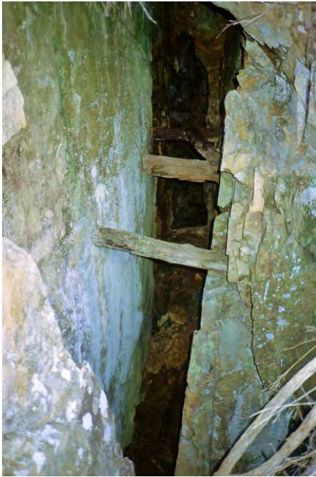
Shafts – shape reflects the narrow width of the quartz vein being mined (D Scott 1985)
