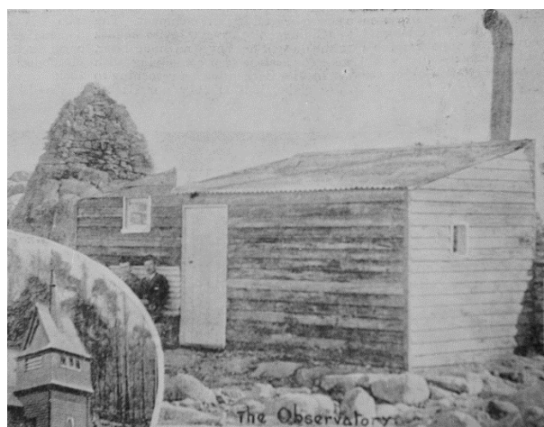
Fig 15. Observatory hut with north wall clad in weatherboards c1896-97, Tasmanian Mail Christmas Supplement 17 Dec 1898, piii
